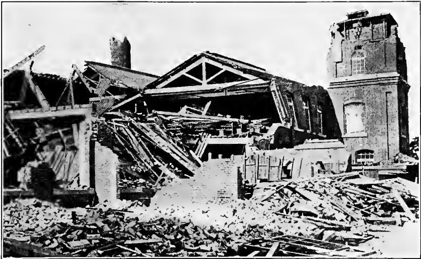
FIG. 281. — Building destroyed by one of the Japanese earthquakes.
